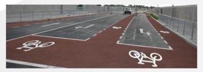
The product detailed in this data sheet forms one of a series of specially formulated high friction road surfacing binders for use with 1–3mm hardened red stone with a Polished Stone Value of 55. The system comprises of two liquid reactive components of moderate viscosity and good reactivity to optimise processing and throughput.
